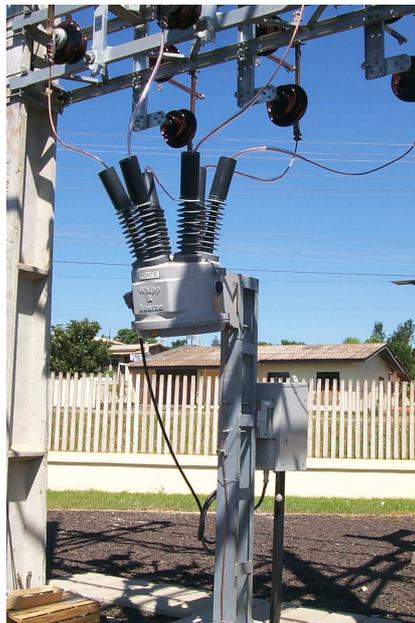
**Figura 9 –Religador Whipp&Bourne com relé Microprocessado SEL 351P (Amazon)**
