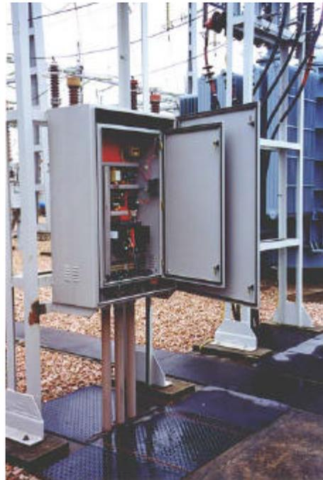
FIGURA 1 – UAD DO TRANSFORMADOR.
