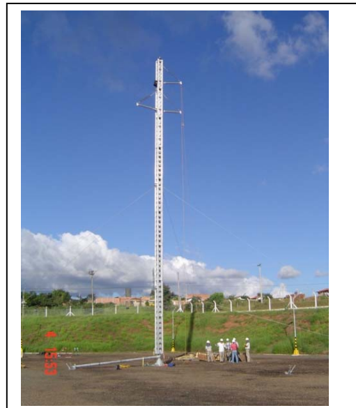
FIGURA 11 – Torre de alumínio 138 kV (Towersolutions)
