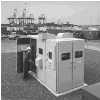
Fig. 7 – Typical Adaptive VAR Compensator Installation
