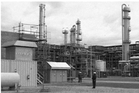
Fig. 4 – Typical Outdoor UPS Installation at Chemical Manufacturer
