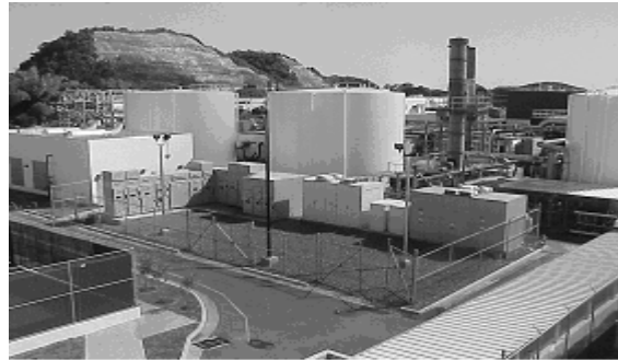
Fig. 12 – Medium Voltage UPS at a Pharmaceutical Plant in Puerto Rico
