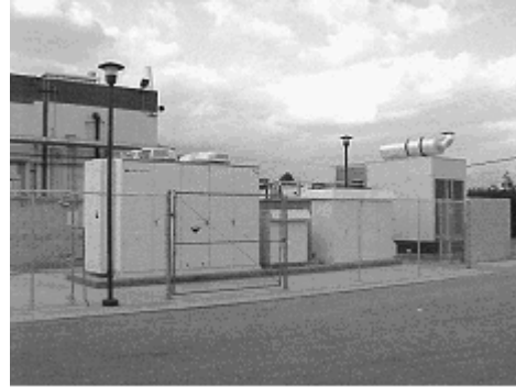
Fig. 5 – Outdoor UPS with Back-Up Generator
