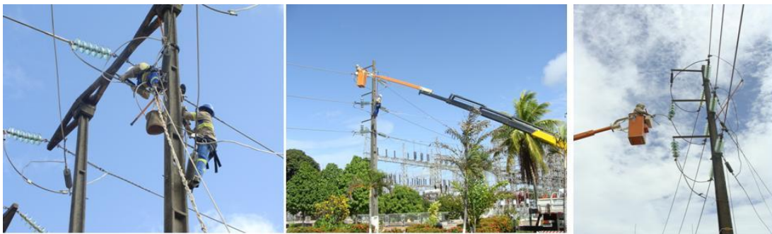
Figura 12 – Conexões com as LT's existentes
